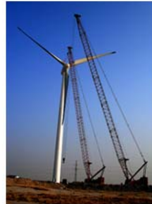
Erection of Changling wind farm
